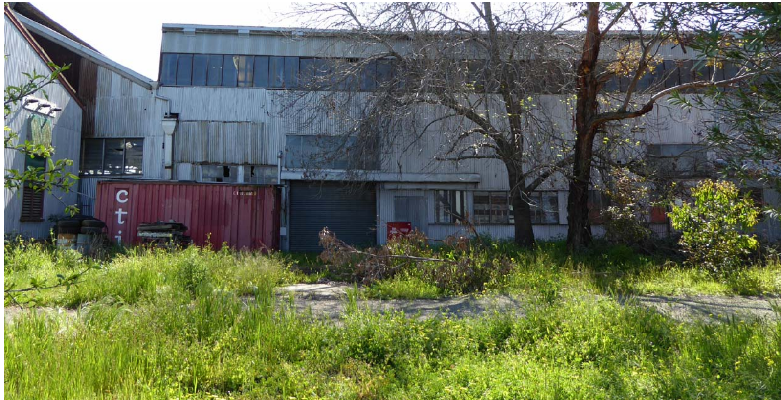
P-02 - BOILER SHOP EXTENSION + MOTOR YARD
