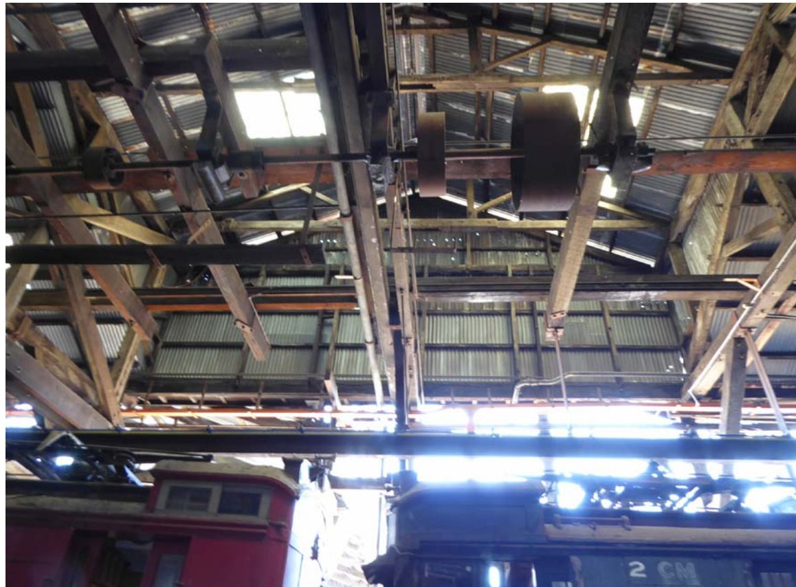
P-02 - FITTING SHOP (WILLIAMSTOWN EXTENSION)
