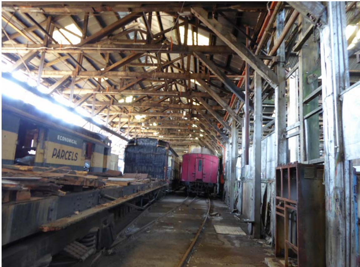
P-01 - FITTING SHOP (WILLIAMSTOWN EXTENSION)
