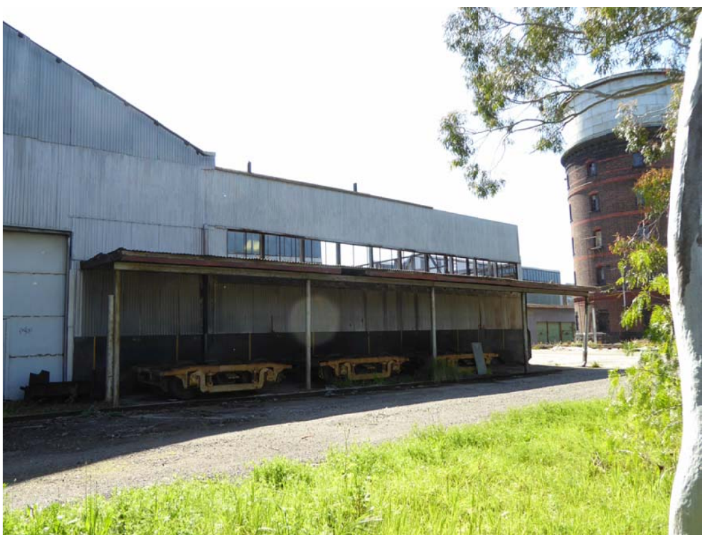
P-06 - MACHINE SHOP EXTENSION
