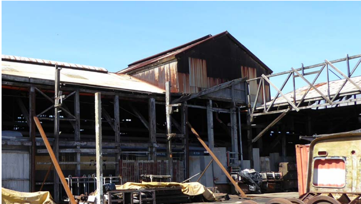
P-03 - FITTING SHOP (WILLIAMSTOWN EXTENSION)
