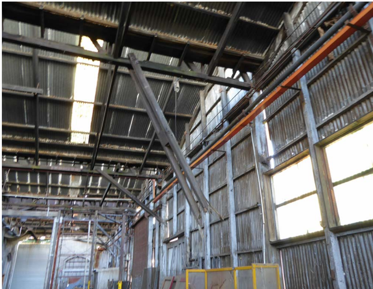
P-04 - MACHINE SHOP EXTENSION
