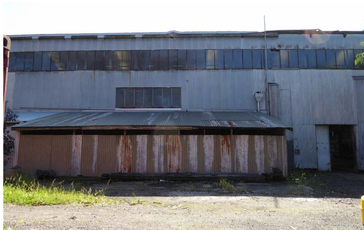
P-04 - MOTOR YARD
