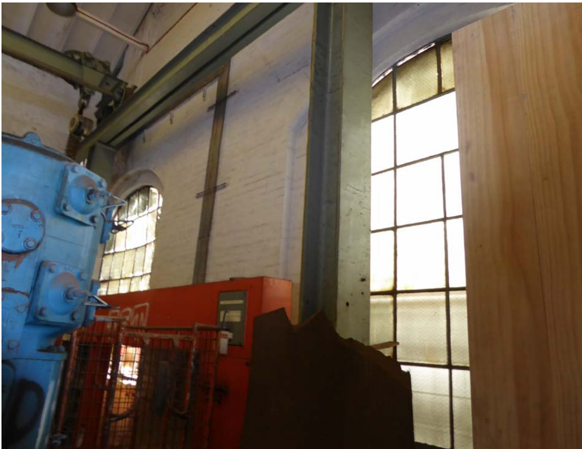
P-07 - EAST ENGINE ROOM (INTERNAL)
