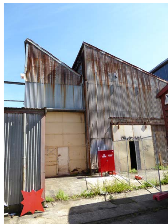
P-01 - MACHINE SHOP EXTENSION
