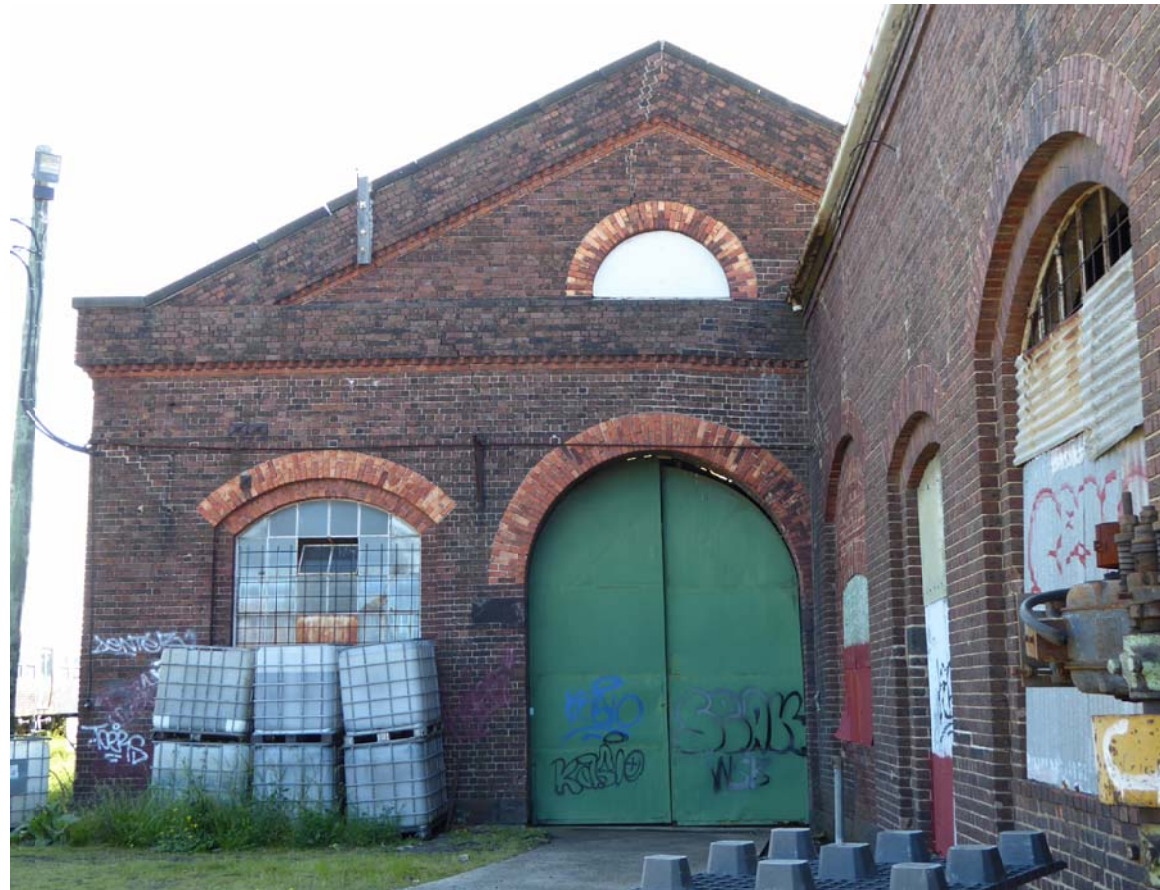
P-01 - WEST BLOCK (SOUTH WEST CORNER)
