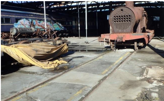
Concrete floor and tracks in the Truck Building Yard
