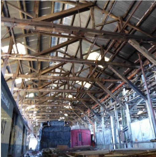
Interior, showing roof trusses
