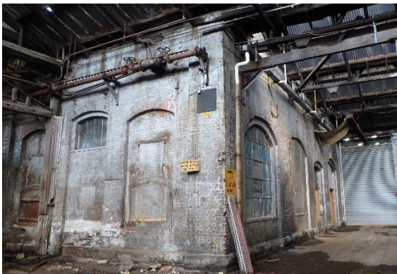
East Engine House, south and east elevations
