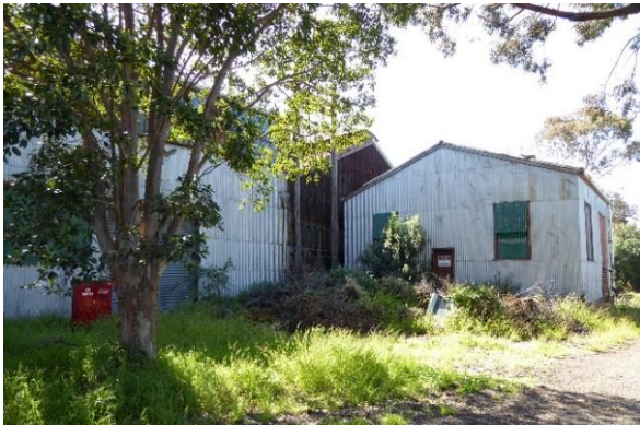
Gable roofed shed
