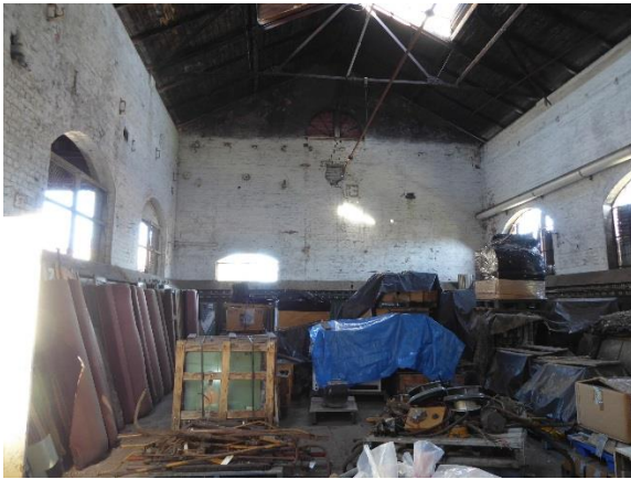
Interior of West Engine House
