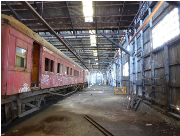
Interior, looking north
