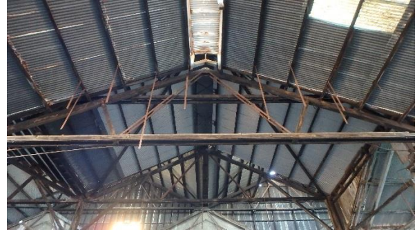
The roof structure
