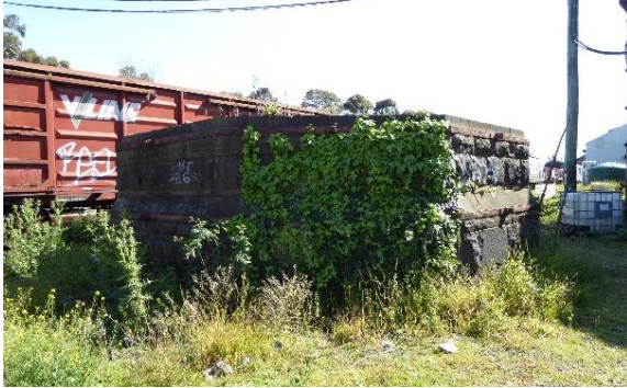
Remnant basalt base of chimney
