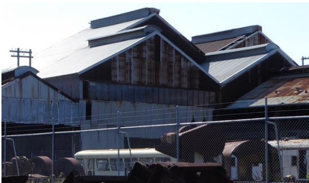
View of Hydraulic Riveter Shop + South of Hydraulic Riveter Shop roof forms from west
