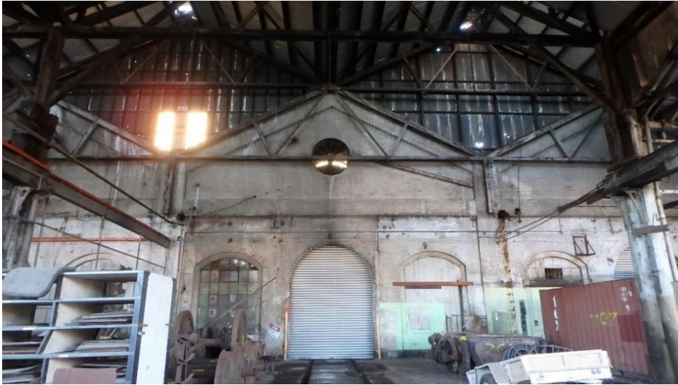
Section of the West Block South Wall, view from within the Hydraulic Riveters Shop.
