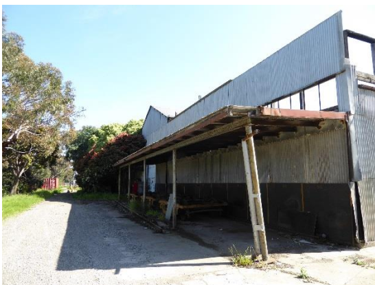
Flat roofed shelter
