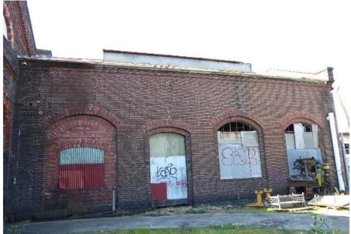
West Engine House, west elevation
