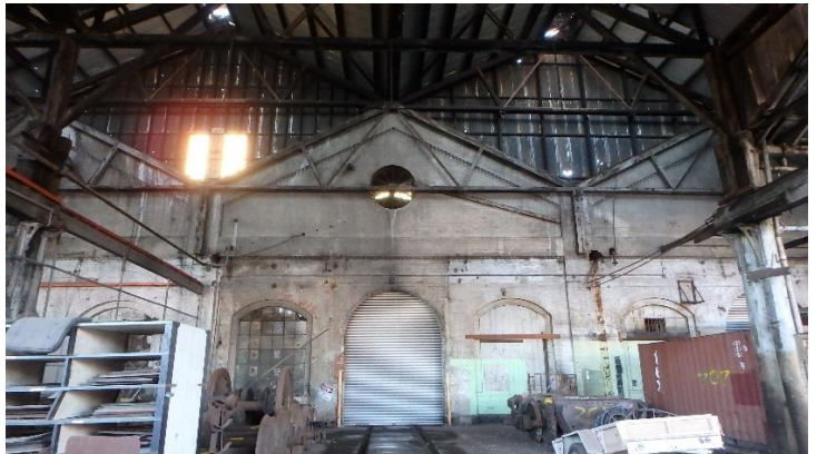
Proposed Partial Demolition, Conservation and Securing Works West Block Southern Extension and West Block (Part), Newport
