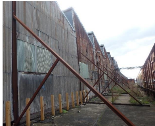
East external elevation
