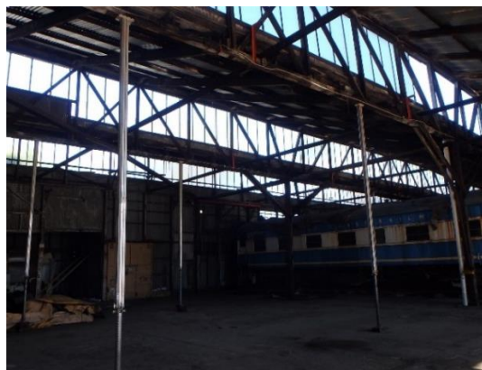
Propping, Truck Building Yard
