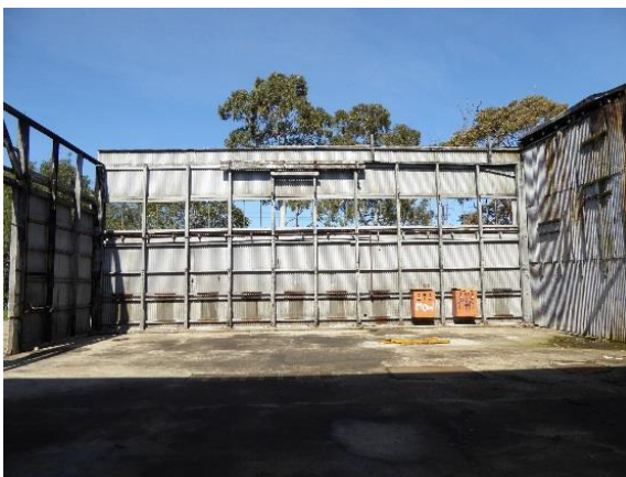
Garage interior, looking south
