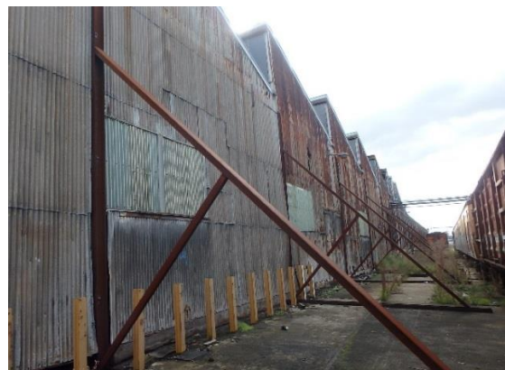
Bracing, east side of Machine Shop Extension
