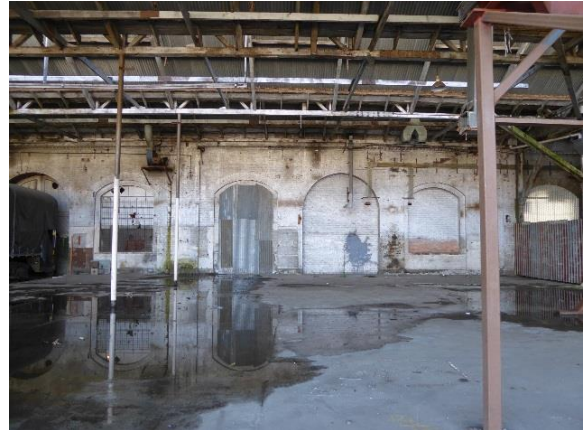
Looking north towards the south brick wall of West Block
