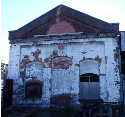
West Engine House, south elevation
