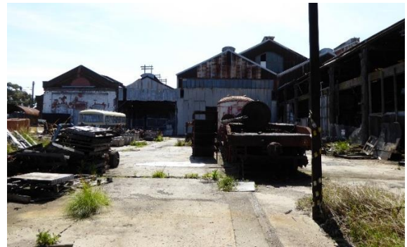
Area of concrete to the west
