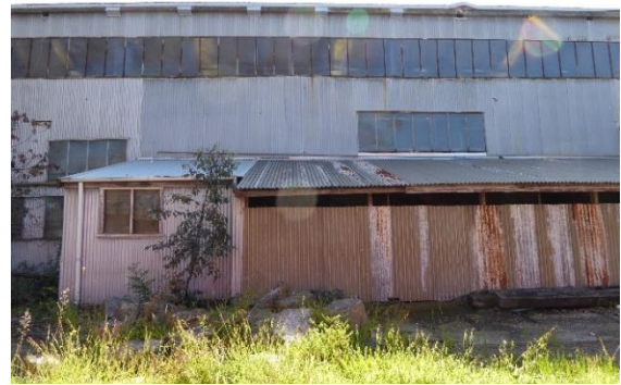
Skillion roof shed
